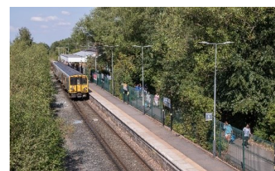
Ormskirk rail station
